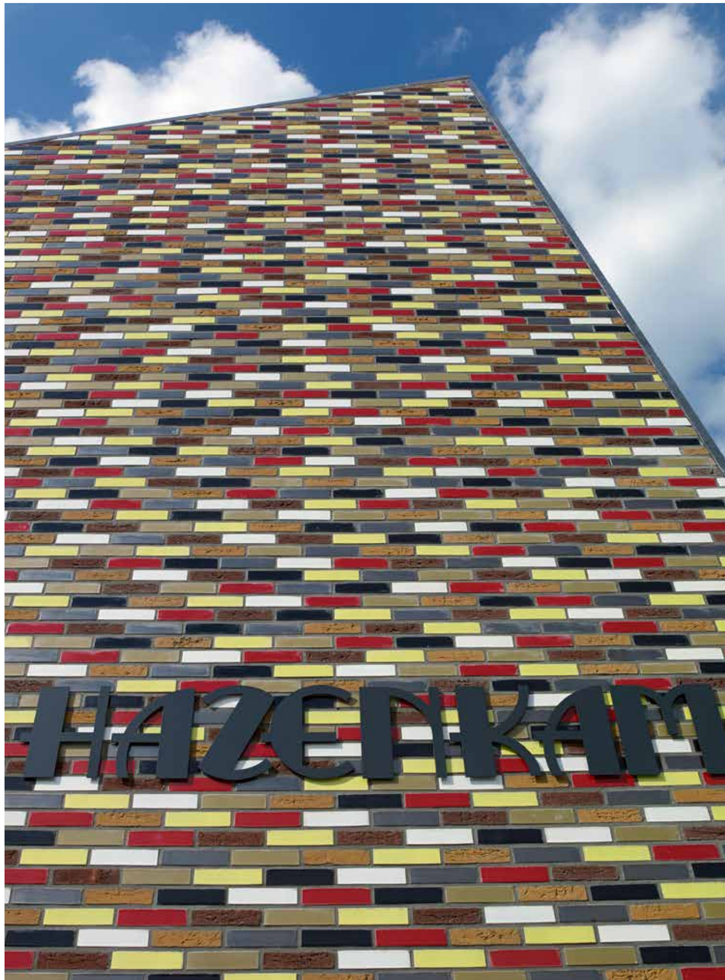
Mix of glazed bricks
