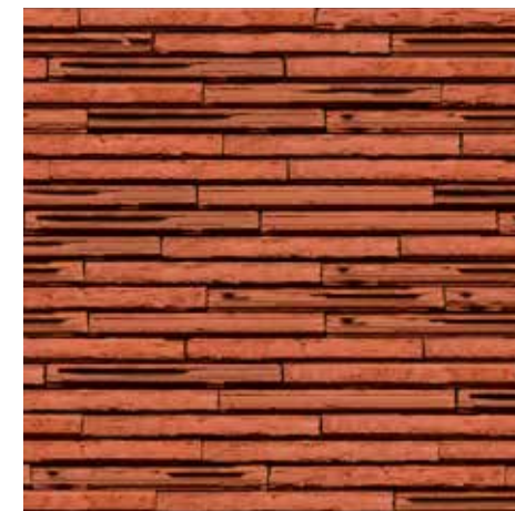
Mixed appearance (laid so that a mixture of smoothed and broken stretchers is showing)
