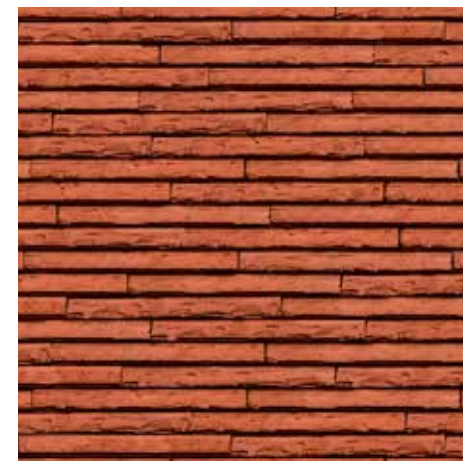
Purely smoothed appearance (laid so that only the smoothed stretchers are showing)
