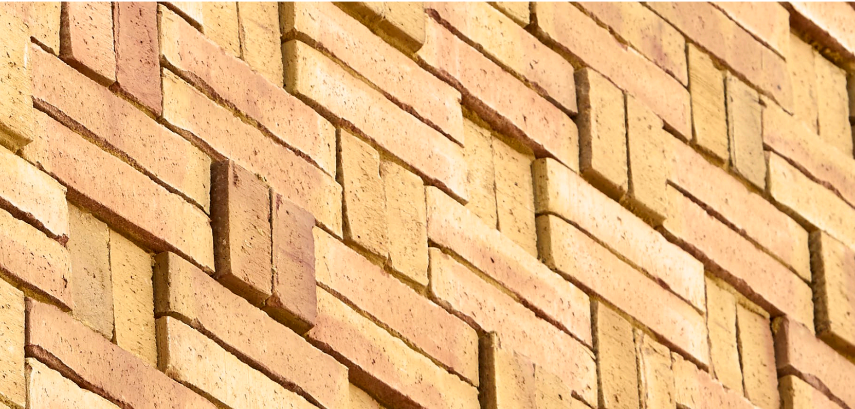
Flemish bond of double stretchers and headers
